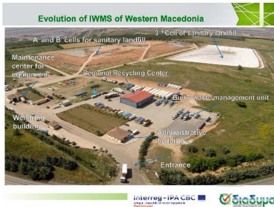
Figure 21. Facility for the IWMS, DIADYMA S.A., Greece
